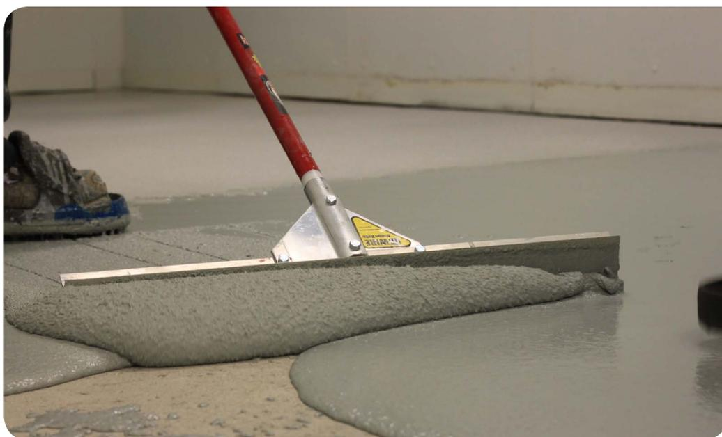
systems, protective and marine coatings, roof coatings, and decorative concrete products. Application squeegees are typically used to spread and disperse coatings at thinner film builds — less than 60 mils (1,524.0 microns).
